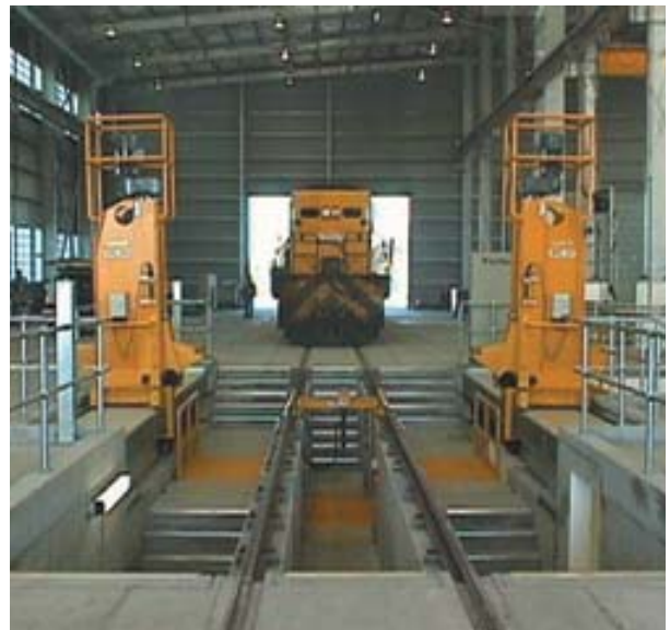
New drop table at Redbank, Queensland.
