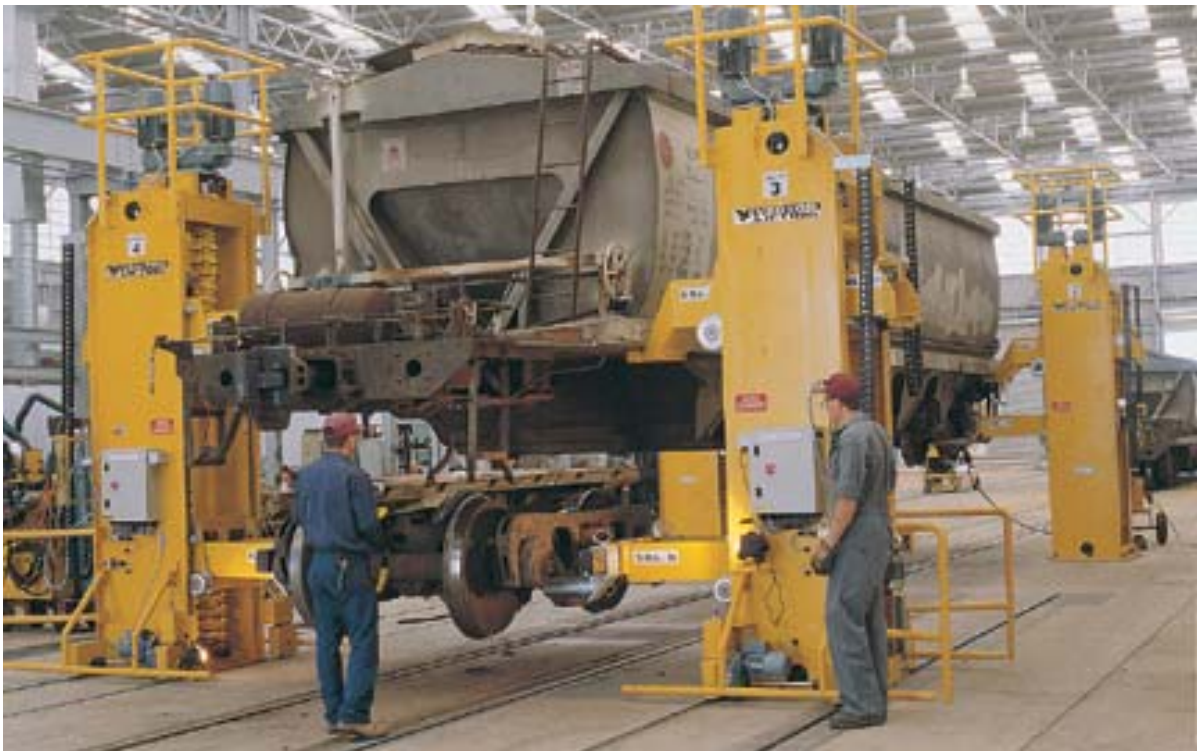
Vectors's new Double Lifting Jack System facilitates repair and maintenance at the Willowburn Wagon Maintenance Depot, Queensland.
