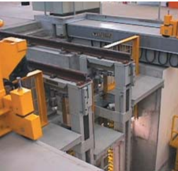
View into the drop table pit at Redbank, Queensland.
