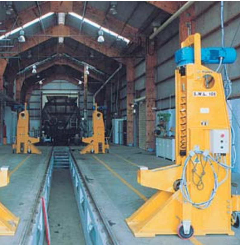
Wagon repair depot with 10 tonne jacks in position at Albany, W.A.
