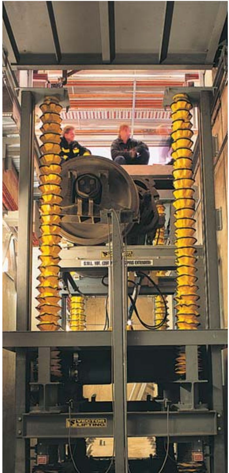
Above: A wheel set on the drop table photographed from inside the travel pit area at Spotswood, Victoria. Left: One of Melbourne Trams famous vehicles being prepared for maintenance, elevated on Vector's under floor lifting system at the Preston (Vic) workshop.
