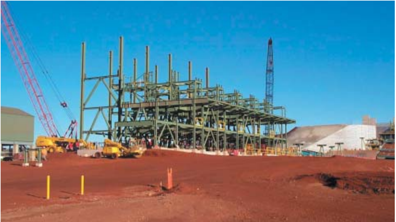
Above: West Angelas minesite Screen Building.
