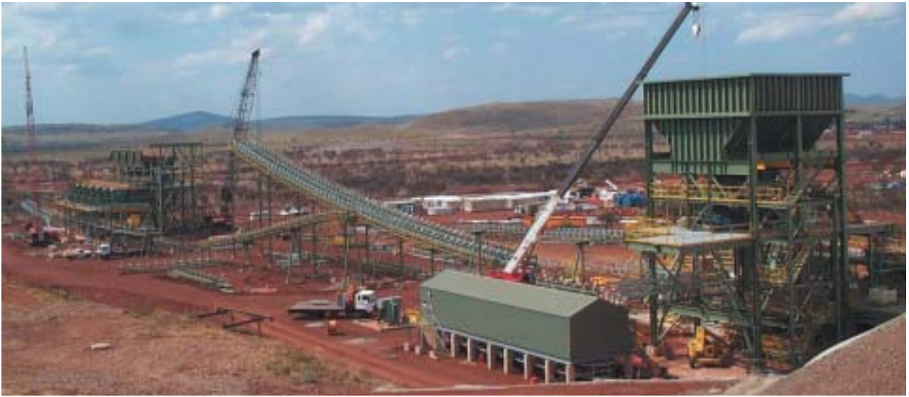
West Angelas minesite Secondary Crush Building.
